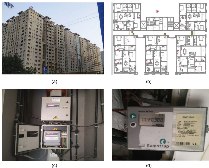
Fig. 2 a Residential complex b Typical floor plan of the buildings c Energy meter d BTU meter
